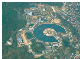
Uegahara Purification Plant (Nishinomiya City) capacity: (Rapid filtration) 70,000 m 3 /day
